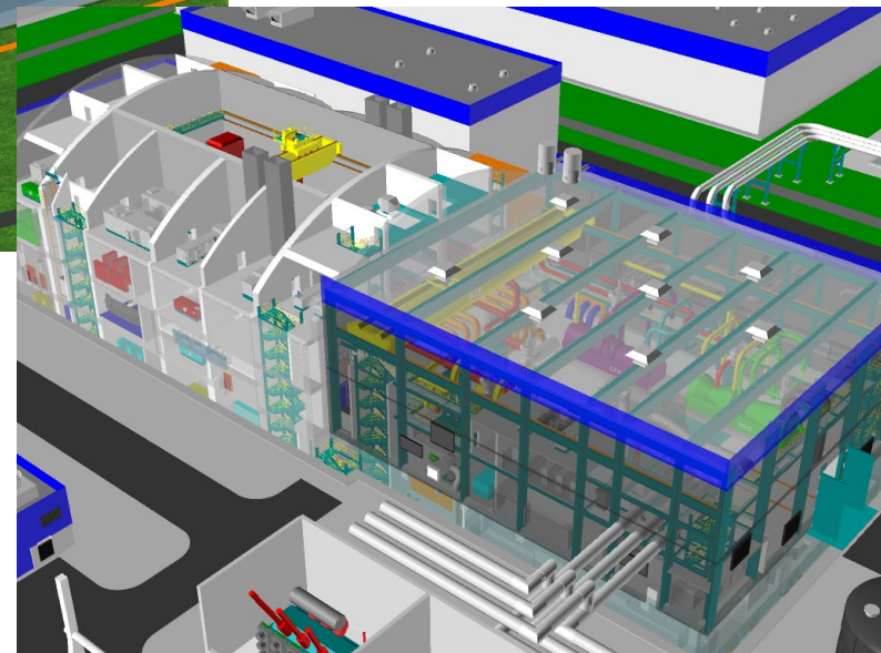
Nuclear Island and Turbine Building
